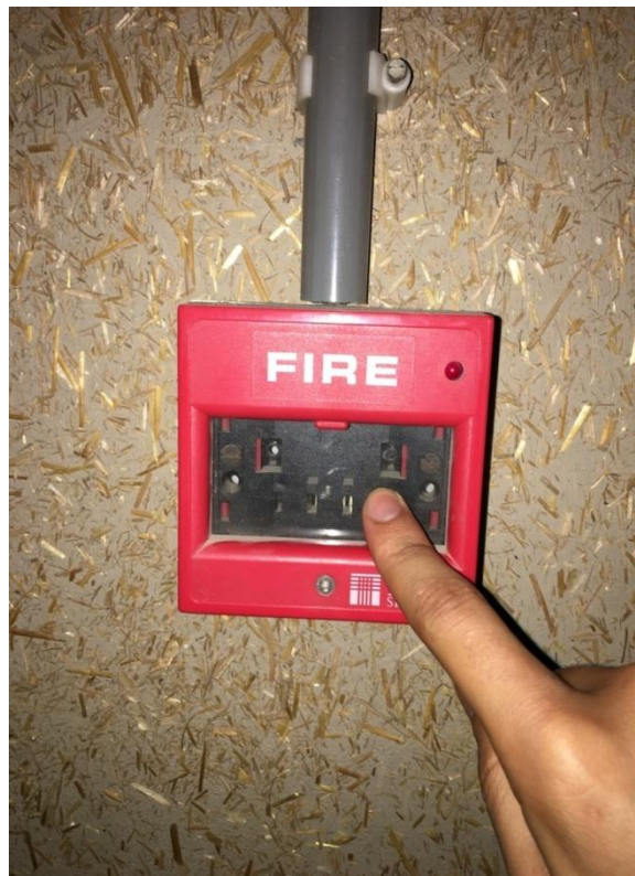
Fig.14 Manual glass breakers are not working (Source: by Researcher)
