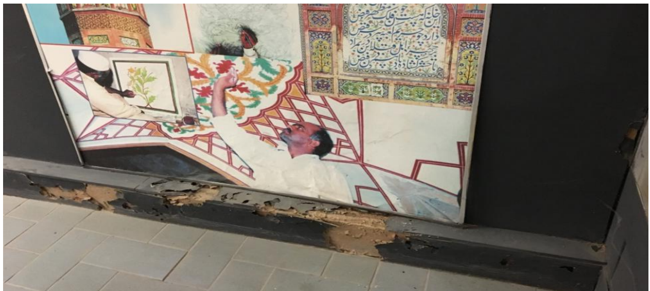
Fig.9 Termites attack on Royal Kingdom of Saudi Arabia internal tent (Source: by Researcher)
