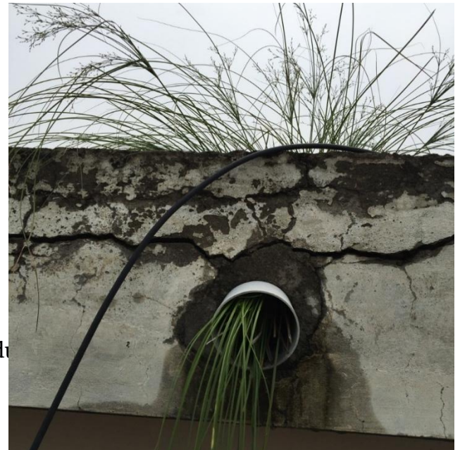
Fig. 7 Water ponding at left side on Roof due to grass growing (Source: by Researcher)
