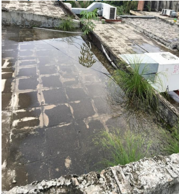
Fig. 7 Water ponding at left side on Roof due to grass growing (Source: by Researcher)
