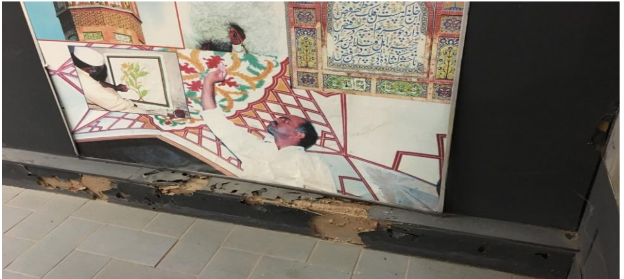
Fig.10 Termites near D-37(Islamic Architectural panel door) (Source: by Researcher)
